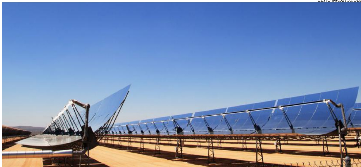
Figure 5. Parabolic trough-type concentrating solar power (22).
