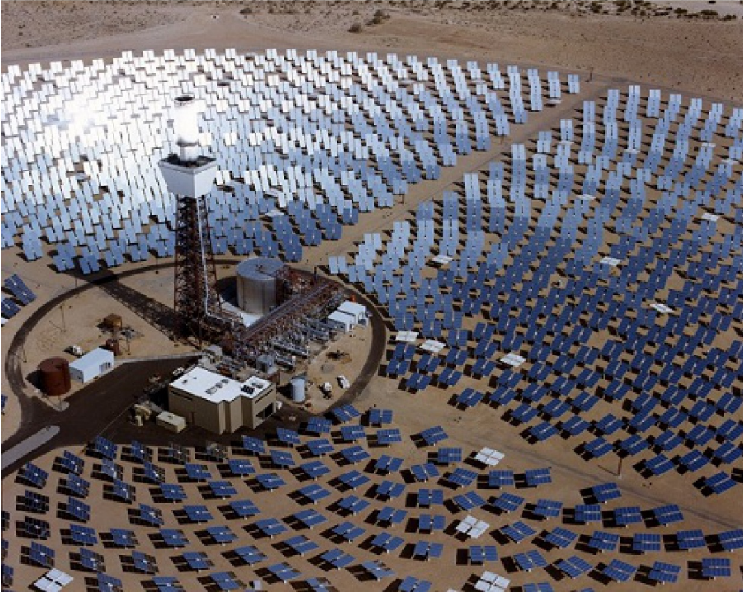
Figure 6. Central receiver-type concentrating solar power (19, 22).
